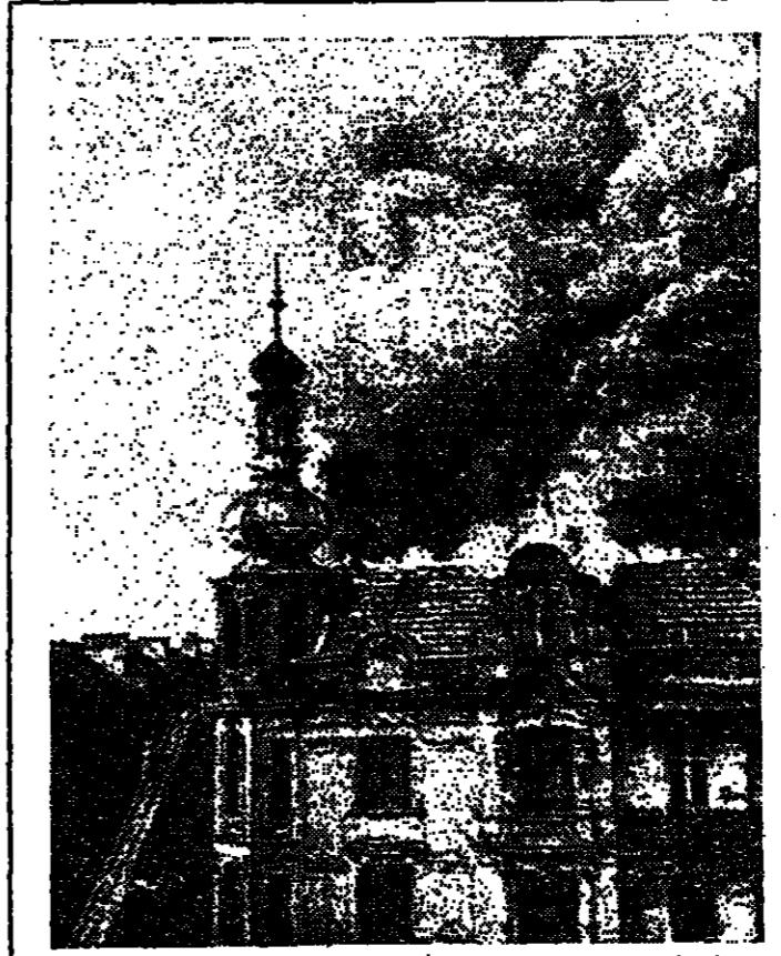
SMOKE OF PAST GLORY—Firemen in Szczecin, Poland, fight a fire in an apartment house where 20 homes were destroyed Monday. The building, now the ruins of a tenement, was once an ornate structure.
